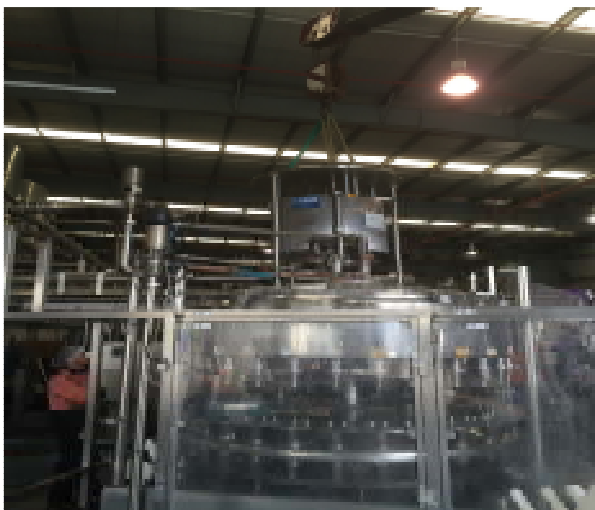
New capping machine being craned into position
